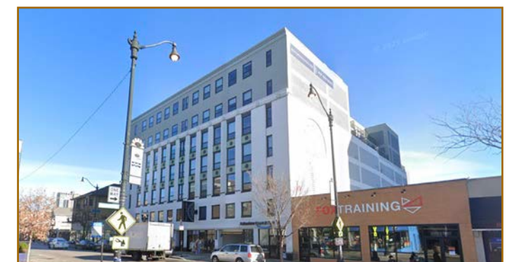
Figure 12- 3121 N. Broadway, Chicago. Credit: Google Street View, 2025
